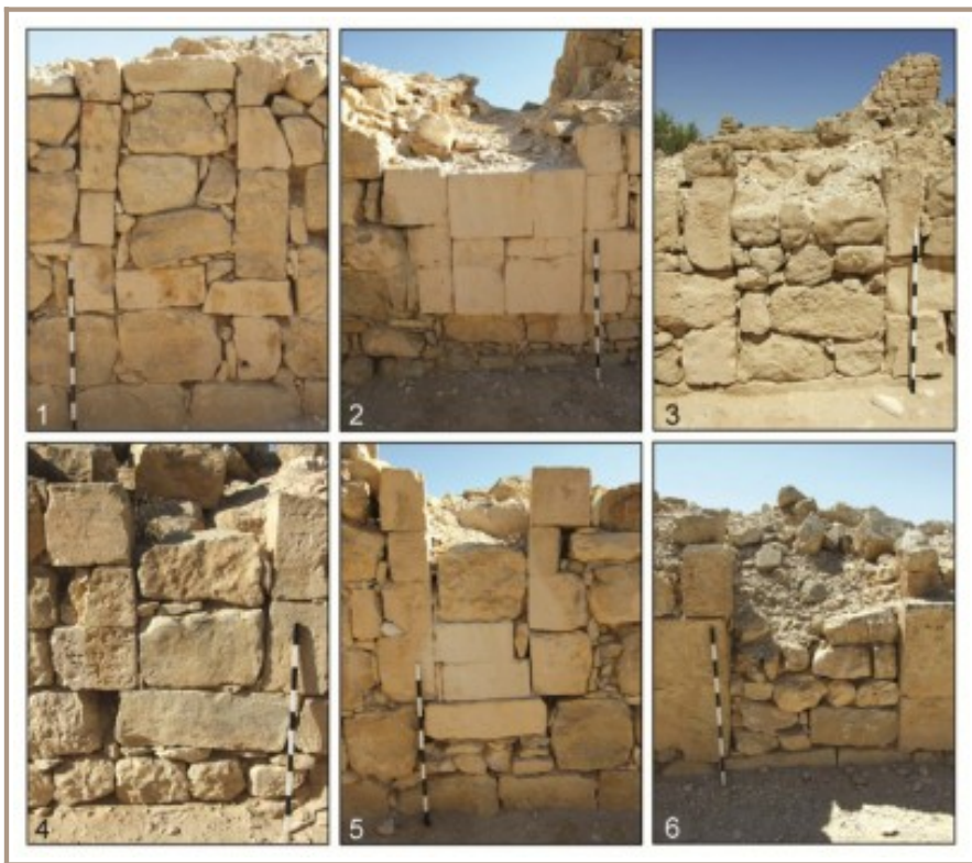
Figure 3. Six examples of sealed door openings at Shivta, including doors that are completely barricaded (1) and others that are sealed using finely dressed masonry (2–5) or small unmodified stones (6).
